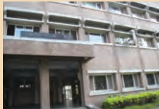
▲ 農機工廠後門 Rear view of AMW
