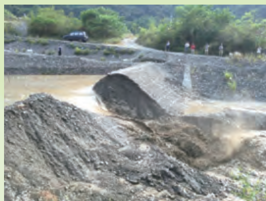
▲上圖為惠蓀林場堰塞壩潰壩試驗場域 The photo shows a landslide dam breaching test in Huisun Forest station
