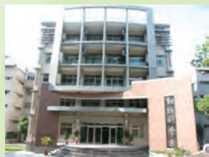
▲動物科學系系館大樓 The building of department of animal science.
